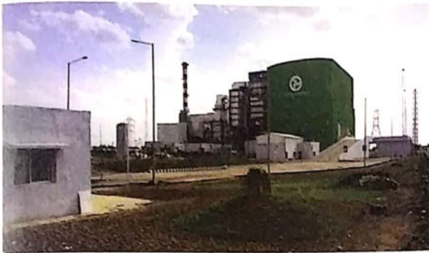
Jabalpur Waste-to-Energy Plant on PPP mode
