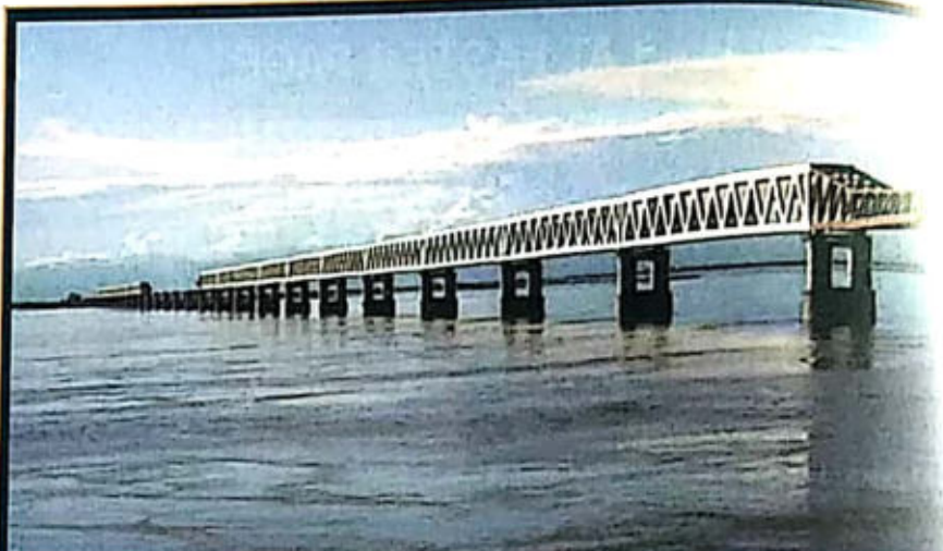
The Bogibeel Bridge, the longest Rail-cum-Road Bridge of the country running 4.94 km in length across river Brahmaputra near Dibrugarh in Assam has been commissioned, connecting Assam and Arunachal Pradesh. Dedicated to the nation by the Prime Minister on 25th December, 2018 the bridge has double line track with three-lane road and 74 km of total railway track.
